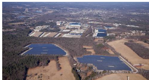
IESI's 8.6 MW project in Franklin MA.
