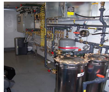
Above are photos of the interior of Remediation system trailers.
